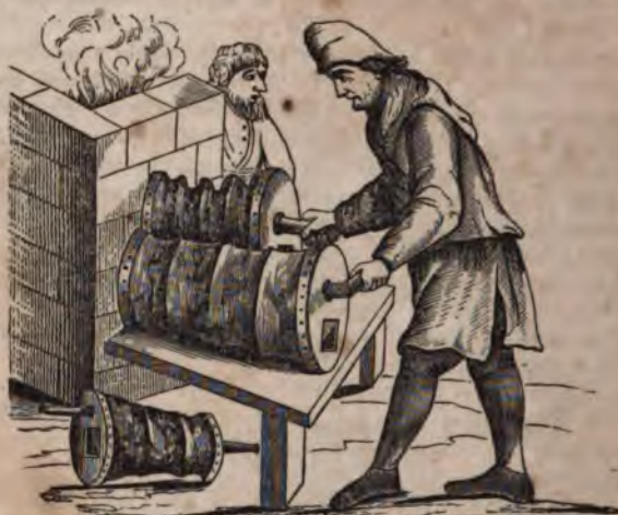
No. 105. Lantern Bellows from Agricola
